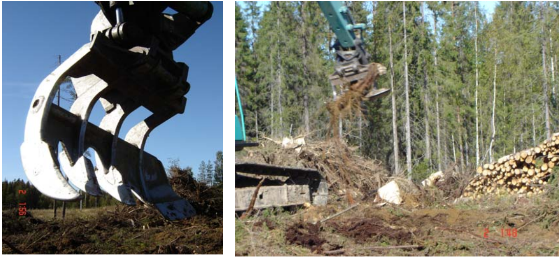
Fig. 3. Stump excavator (left) and stump recovery (right).
